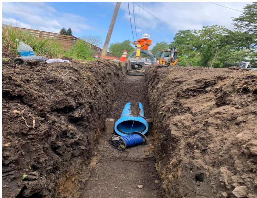
Work continues on Orange Ave Main replacement
