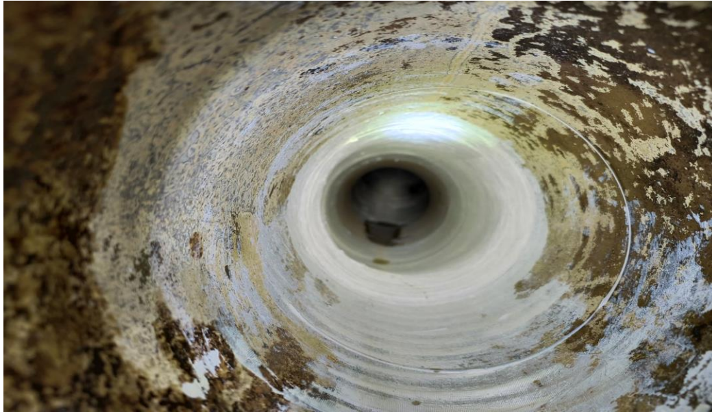
Snap shot of video from Temelec 1 MG lining repair
