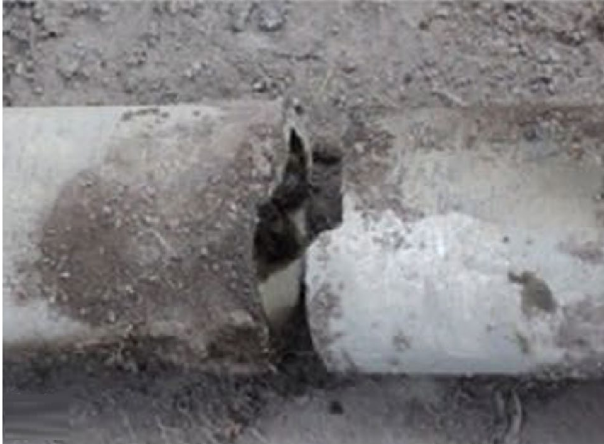
Asbestos Cement (AC)
