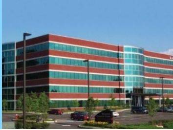
Newterra Corporate Headquarters 1555 Coraopolis Heights Rd. Suite 4100 Coraopolis, PA 15108 USA
